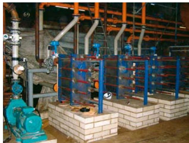
Alfa Laval DIABON® plate heat exchangers in NS1 material used for cooling carbon steel pickling acid in a German steel plant.
