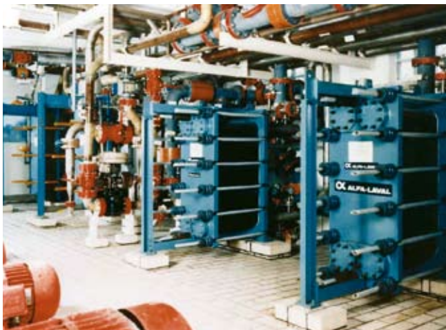
Alfa Laval DIABON® plate heat exchangers in F100 material used for weak sulphuric acid cooling in the mercury recovery section of a Finnish zinc plant.
