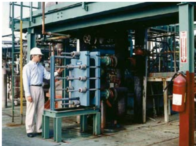
Alfa Laval DIABON® plate heat exchanger in F100 material used for cooling of a mix of hydrochloric acid and chlorinated hydrocarbons in a US plant.
