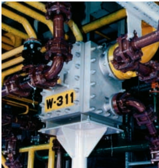
Compabloc assymmetric multipass condenser makes condensation and subcooling possible in the same unit
